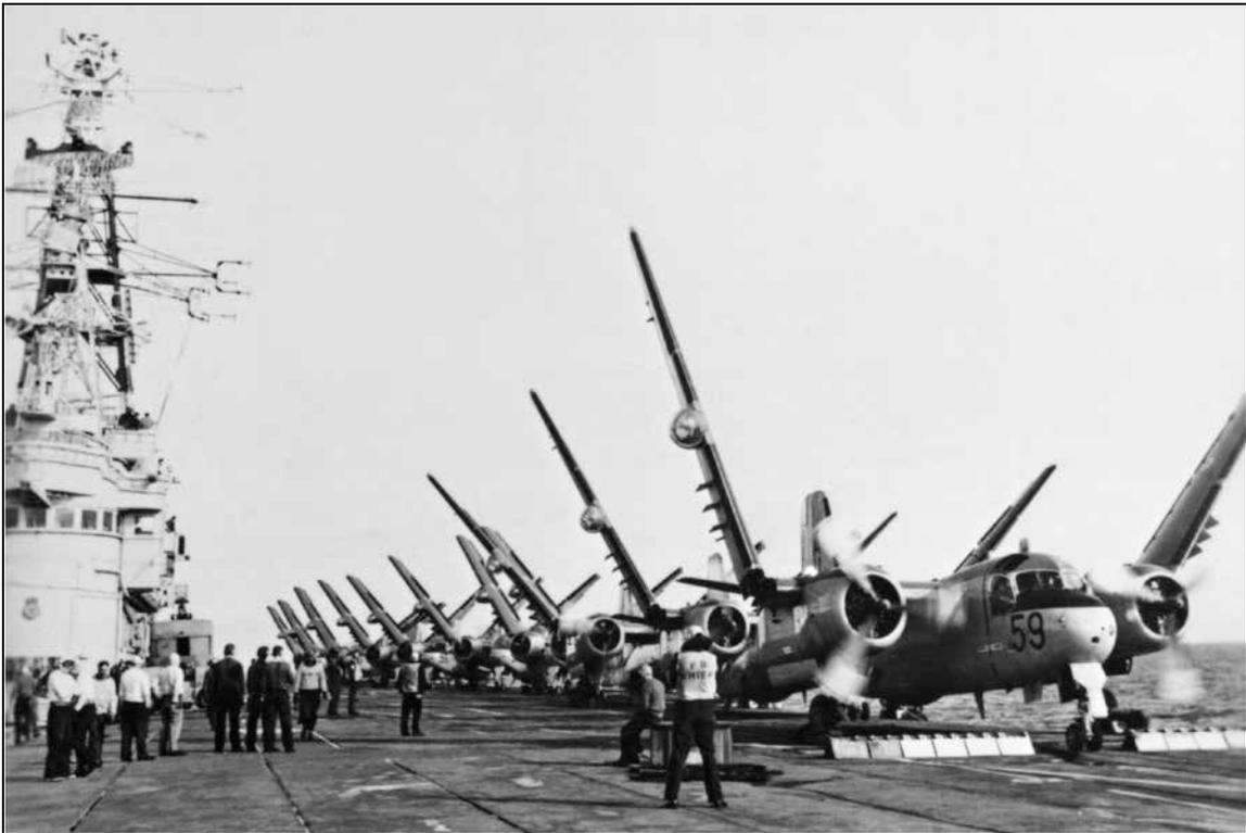
**Ten CS2F-1 Trackers of VS 880 'A' squadron, all with engines running, unfold wings and prepare to launch for an Exercise from the deck of HMCS *Bonaventure* sometime in early 1959. (CAvM Photo 16430)**
